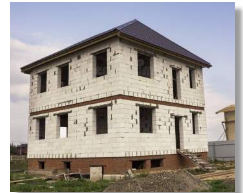
Concrete bricks masonry
