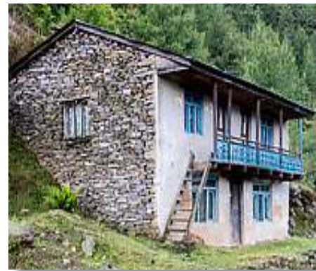
Rubble stone masonry
